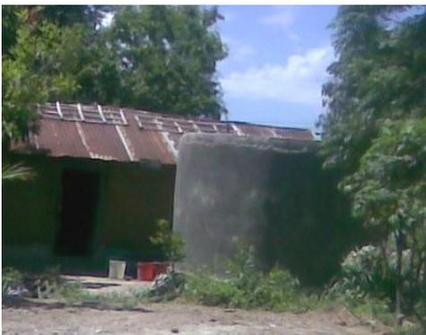
**The Water and Sanitation Project** has almost completed the building of a rain water catchments tank for one of the families. The tank is 3 meters in diameter and will hold 10,000 litres of water. Currently the family rely on a communal tap shared with over 100 other families which flows, at best, for 3 hours out of every 48 hours.
